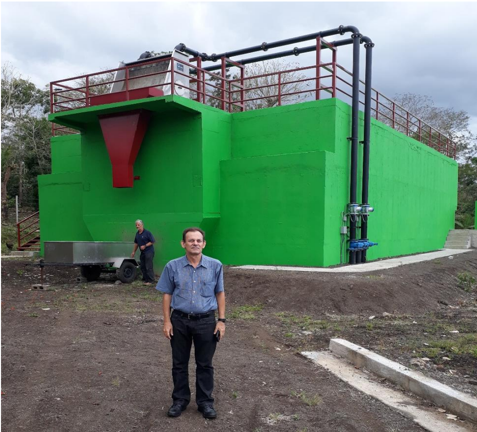
Anaerobic Upflow Reactor (UASB) in La Dalia, Nicaragua
